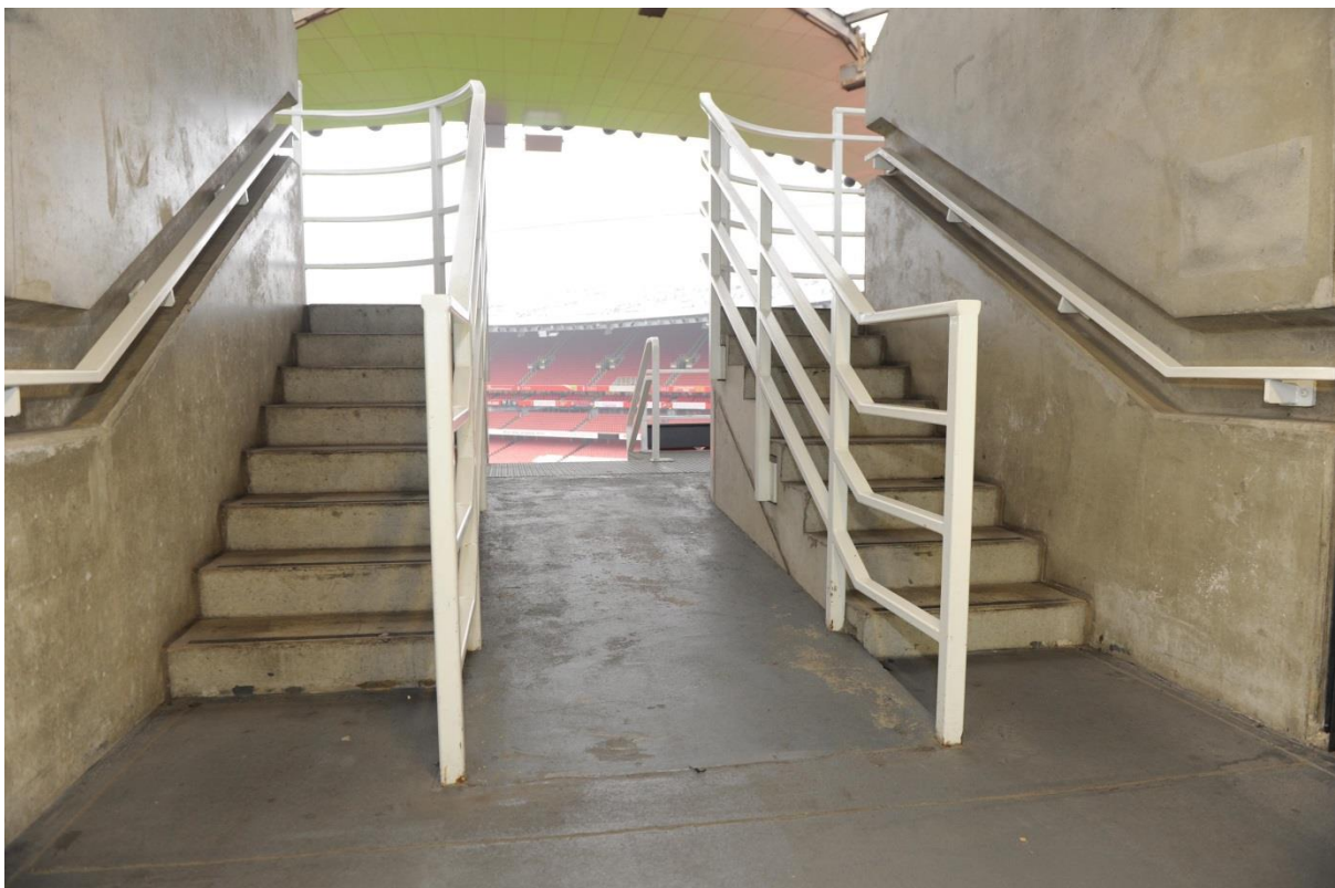
Ramped Entrance to Upper Tier Wheelchair Platform
